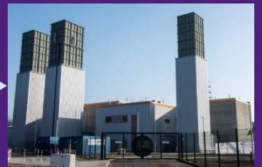
Combustion test center in Berlin
